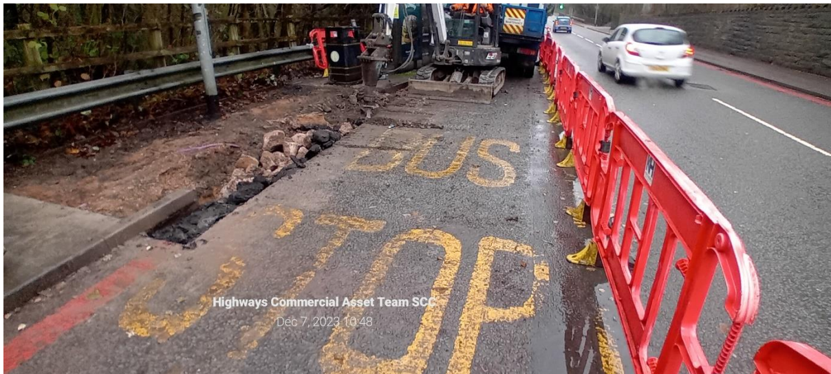
Figure 22 - Bus stop improvement work in progress
