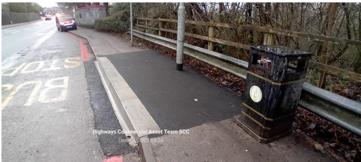
Figure 23 - Bus stop improvement work finished result
